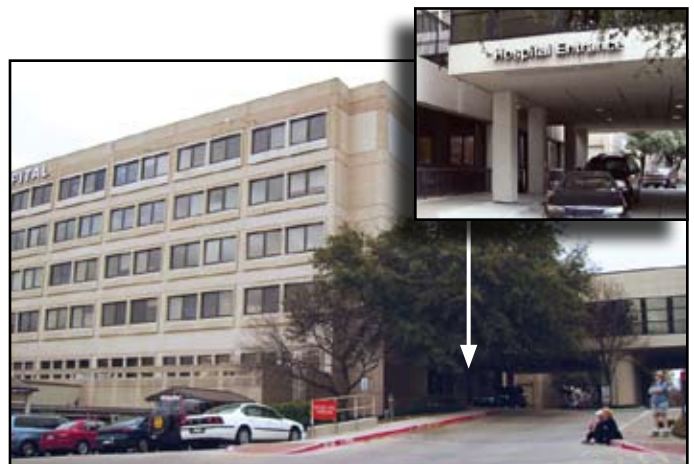
Doctors Hospital from Poppy Drive. The doorway marked "Hospital Entrance" (see inset) leads to the lobby and the Communication Office (Room 112) where the walk box is kept.
